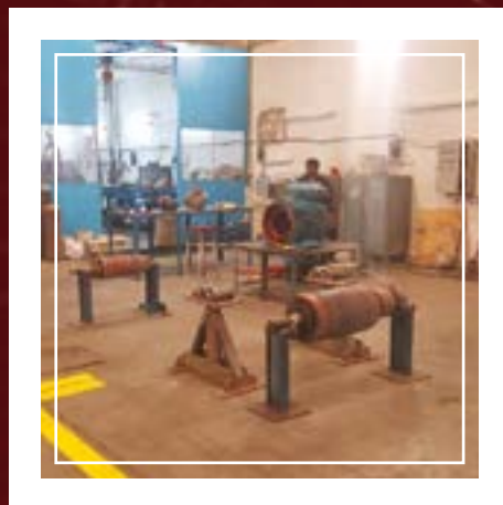
L.T Rewinding Area
